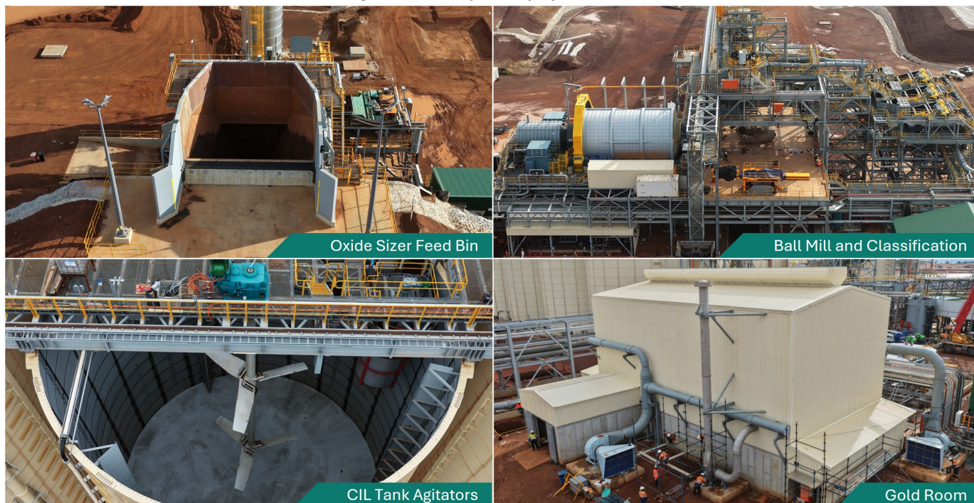
Figure 2: Process plant key infrastructure
