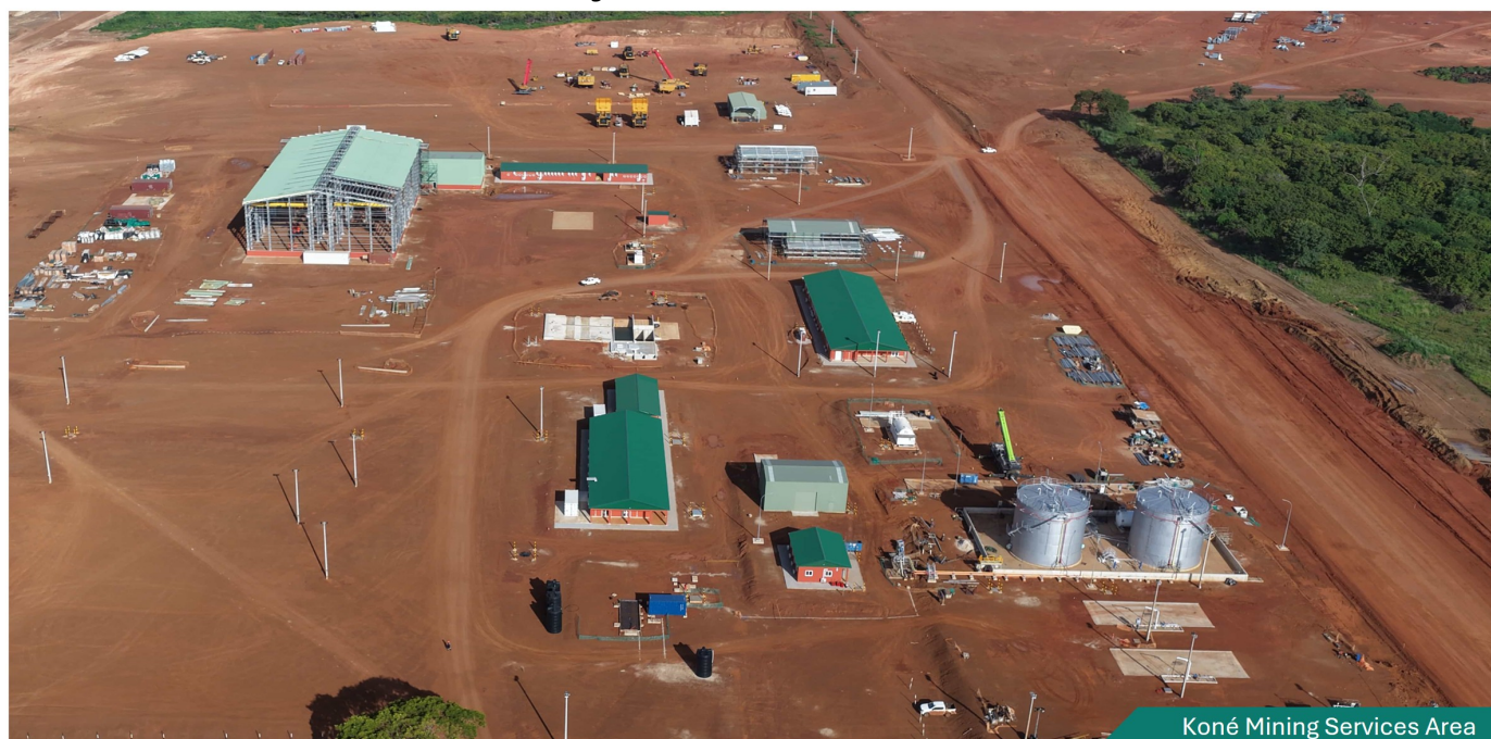
Figure 7: Koné mine services area
