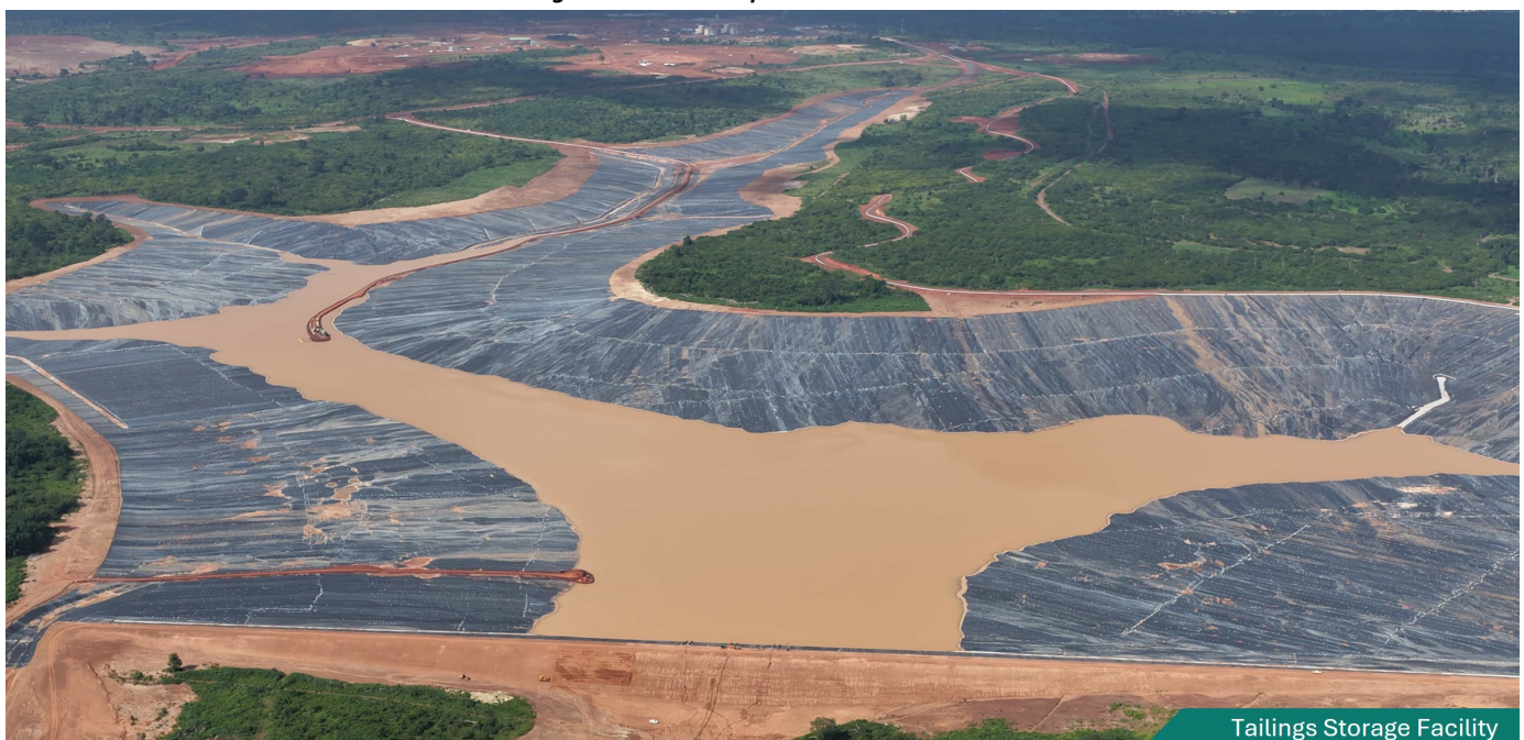
Figure 5: TSF development and HDPE liner
