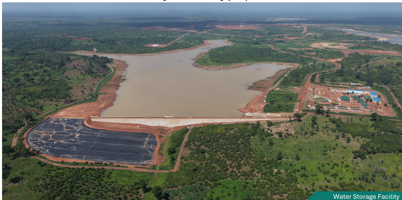
Figure 6: Water storage facility
