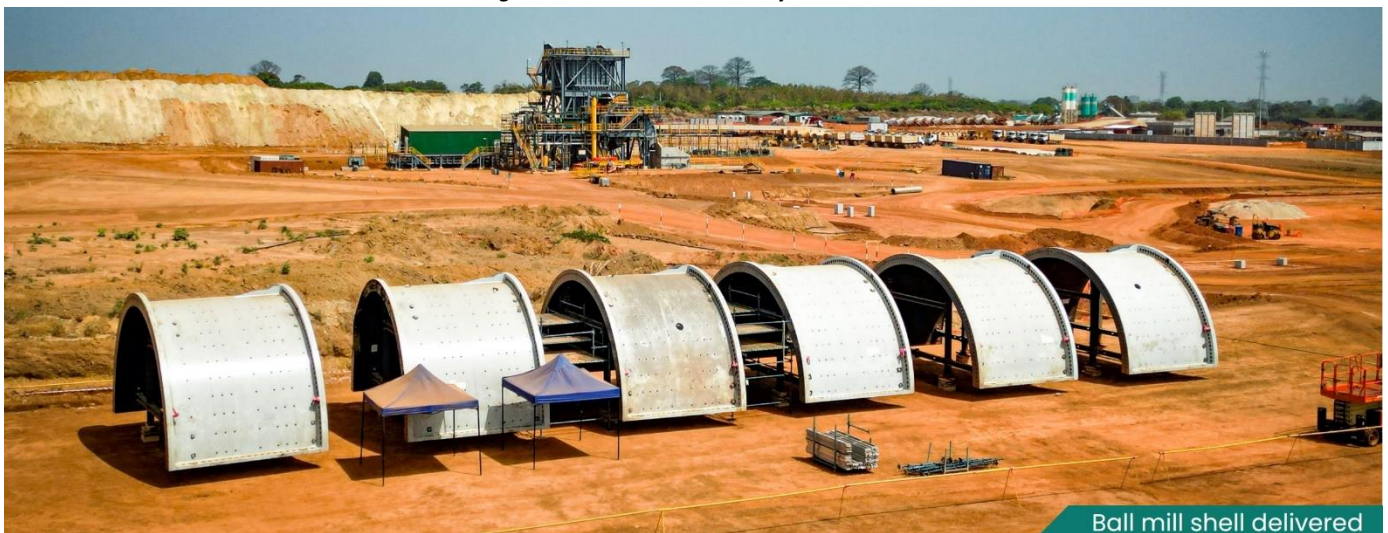
Figure 3: Ball mill shell delivery to site
