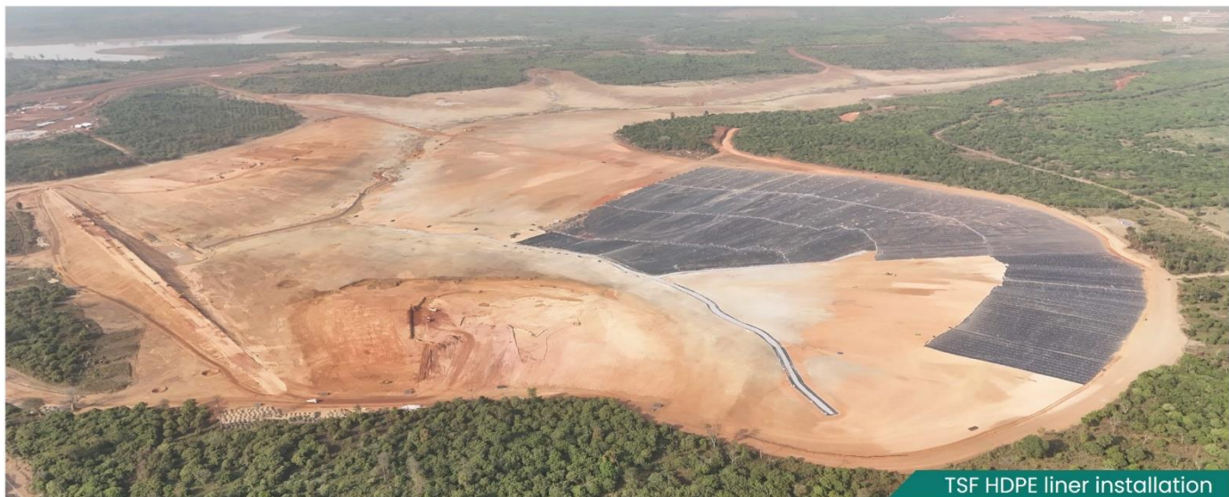
Figure 7: TSF HDPE liner installation
