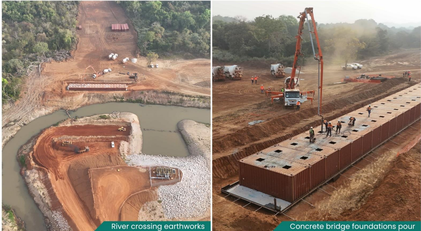
Figure 6: Marahoué river bridge construction
