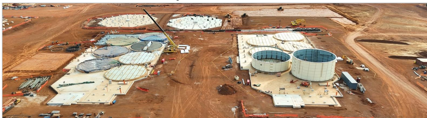
Figure 1: CIL tank installation
