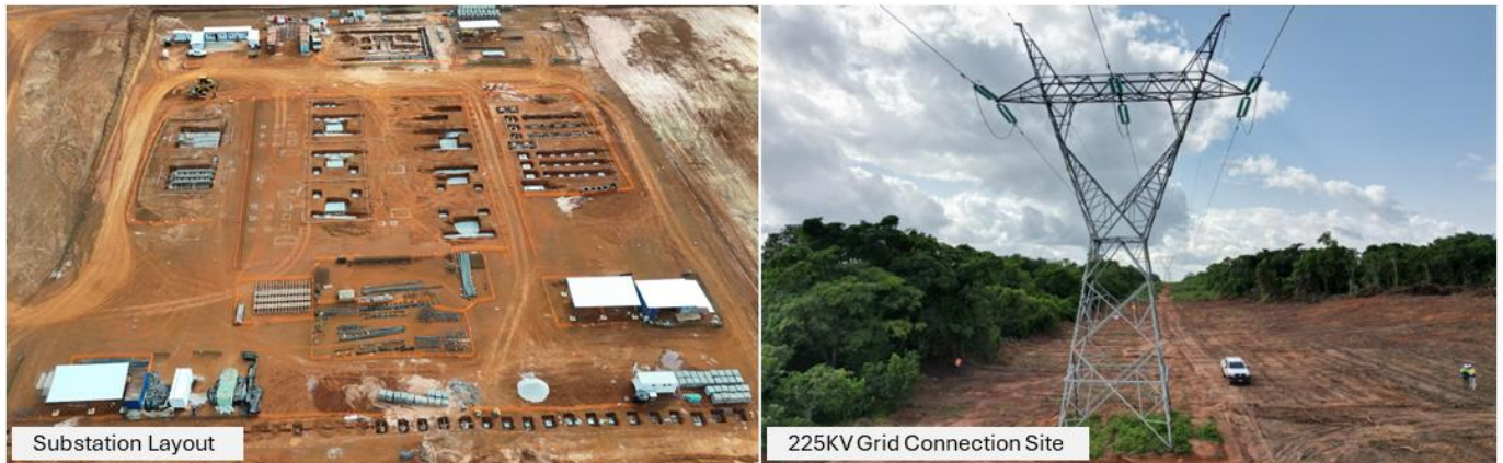
Figure 5: Electrical substation and high-voltage grid connection preparation
