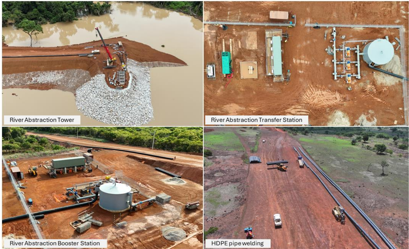
Figure 3: River abstraction site and pumping infrastructure
