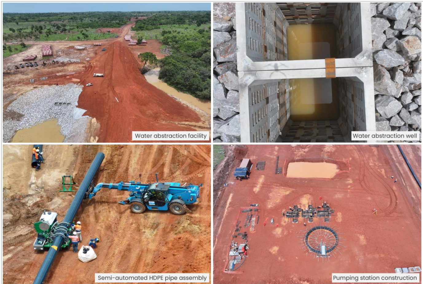
Figure 4: River abstraction site and pumping infrastructure
